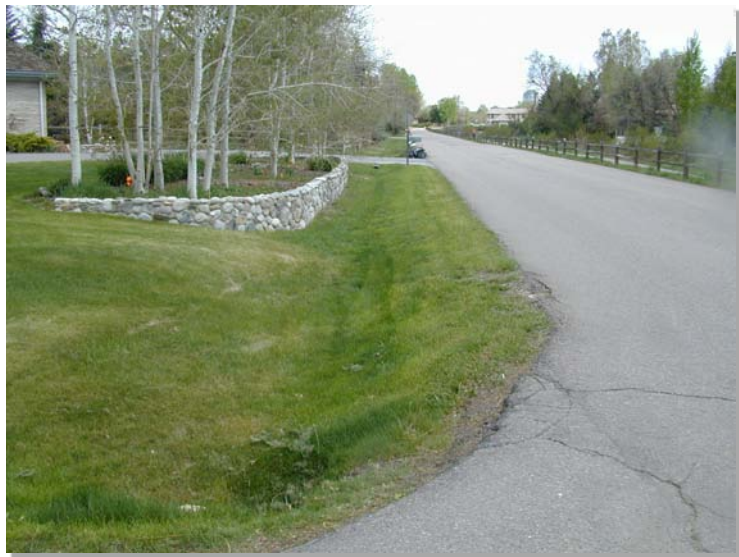
Photograph GS-1. This grass swale provides treatment of roadway runoff in a residential area. Photo courtesy of Bill Ruzzo.
