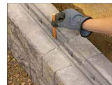
Diagram 6 - Pin Placement (Vertical Channel)
