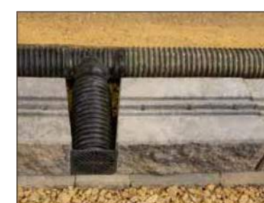
Diagram 7 - Drain Pipe Placement
